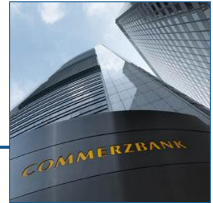
Commerzbank headquarters in Frankfurt.
