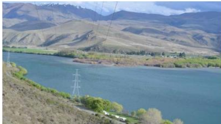
Transmission lines near Transpower's Benmore substation.
