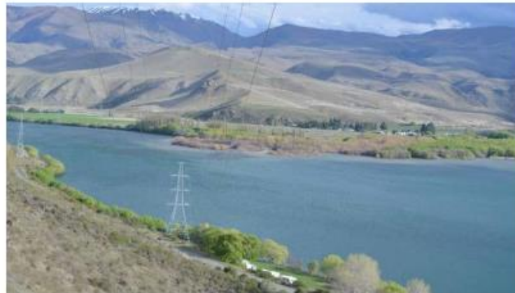
Transmission lines near Transpower's Benmore substation.
