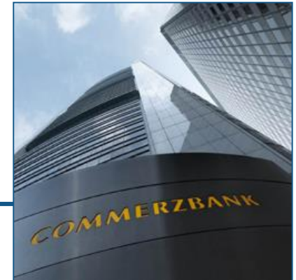
Commerzbank headquarters in Frankfurt.
